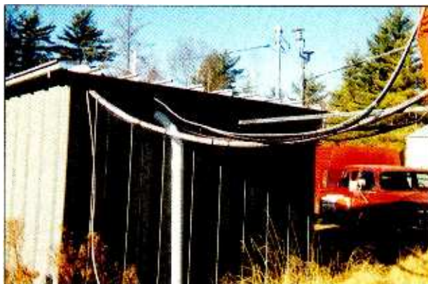
An example of how not to do things. One small ice bridge is used to protect one transmission line. The remaining lines are unsupported and unprotected between the tower and building.
